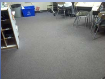
UPHAM: Carpet Replacement in the Modular Classrooms
