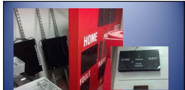
MS: Scoreboard & 30 Second Clock Installation in Gym
