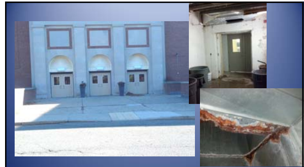
MS: Donizetti Entrance Repairs and Reconstruction
