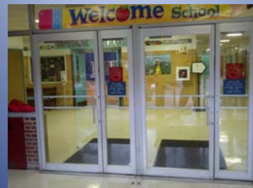
UPHAM: Replace Main Entrance Inner Doors
